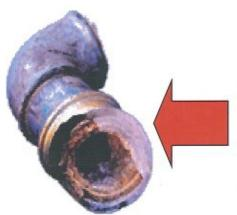
FLUSHING OUR UNIQUE CHEMICAL THROUGH THIS PIPE WILL DISSOLVE ALL ACCUMULATED DEPOSITS WITHOUT HARMING ANY OF THE SYSTEM COMPONENTS.
